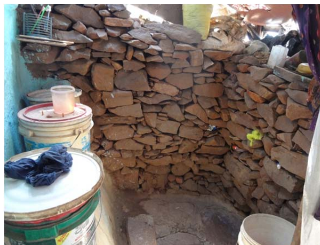
Fig.3: Toilet without a Roof.
